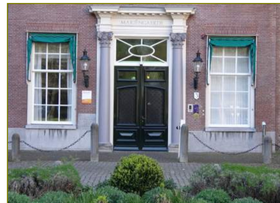
Entree begane grond
