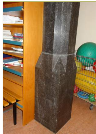
Overgang kolom - basement
